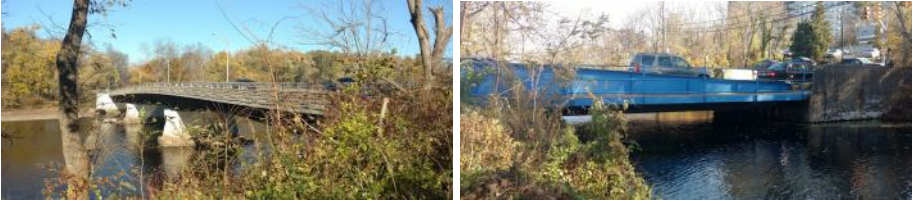
Right: The Landing Lane bridge seen from the entrance to the Delaware and Raritan (DNR) Canal State Park. Left: The now defunct swing arm over the DNR canal.
