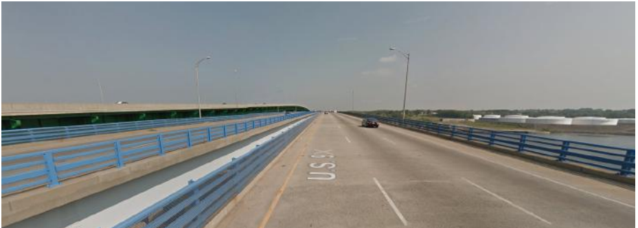
A street level view of US 9 on the northbound side. The new southbound bridge can be seen to the left, and the Driscoll Bridge to the left of that. Photo from Google Maps
